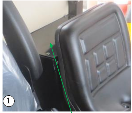
Cover plate of electrical box
